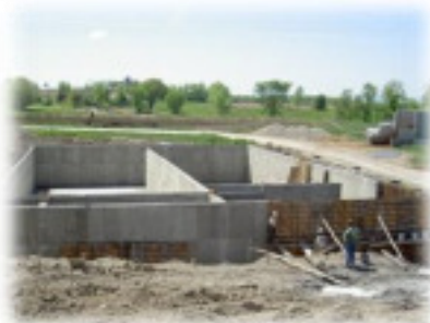
The in-ground vessel retains more heat than above ground
